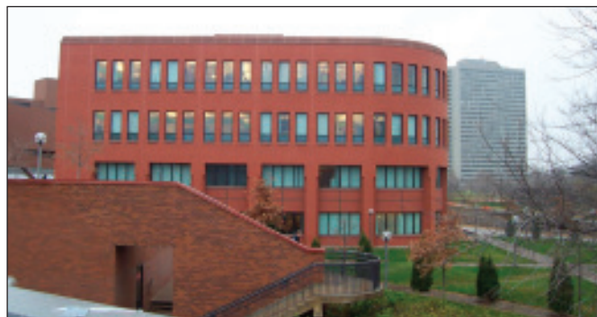
The Andersen Library (above) houses a five-storey, 100,000 square foot lending library above ground and an 84,000 square foot archive facility (cover picture) fifty feet below bedrock. The two facilities are connected by vertical elevator and stair shafts. Structural systems include precast concrete and structural steel.
